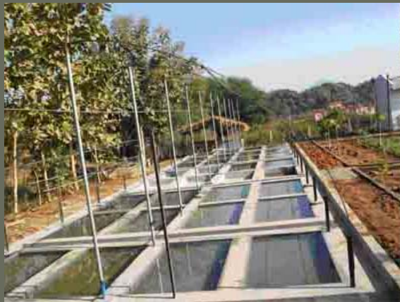
Blue Green Algae (BGA) production unit at Bhawanipatna, Kalahandi (Under Construction)
